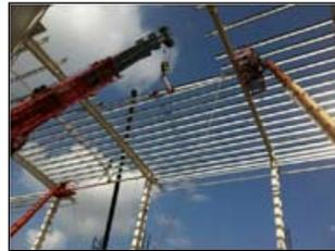
Purlin erection with boom lift and crane
