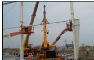
Strut pipe erection by using cranes & two boom lifts
